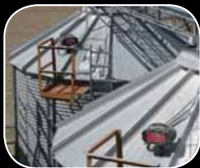
Measuring corn in a grain storage silo.
